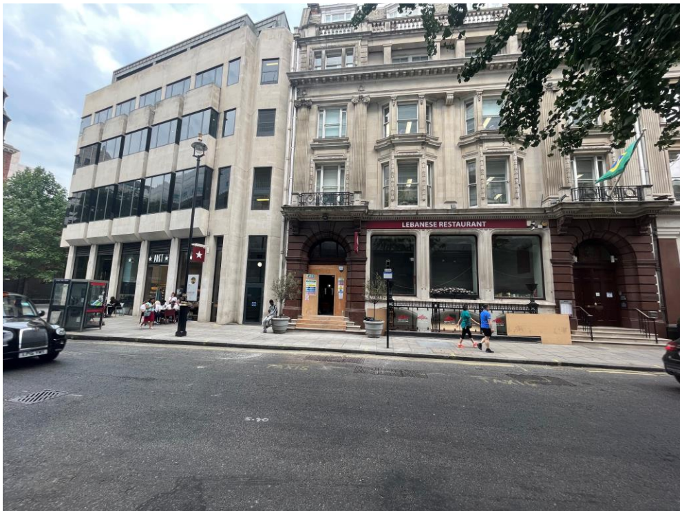
View of 3-4 Vere Street and 1 Chapel Place from the west side of Vere Street
