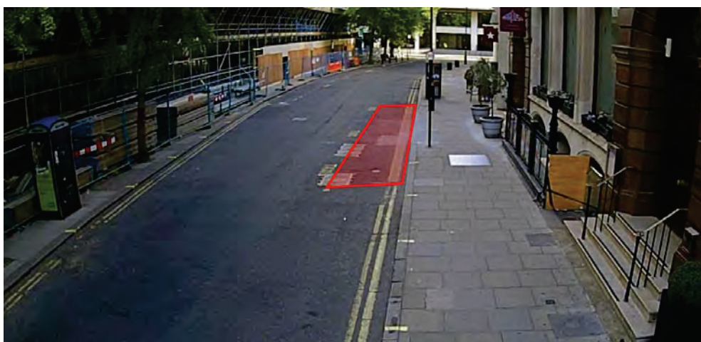
Figure 2.1 – Taxi Bay Location on Vere Street.
